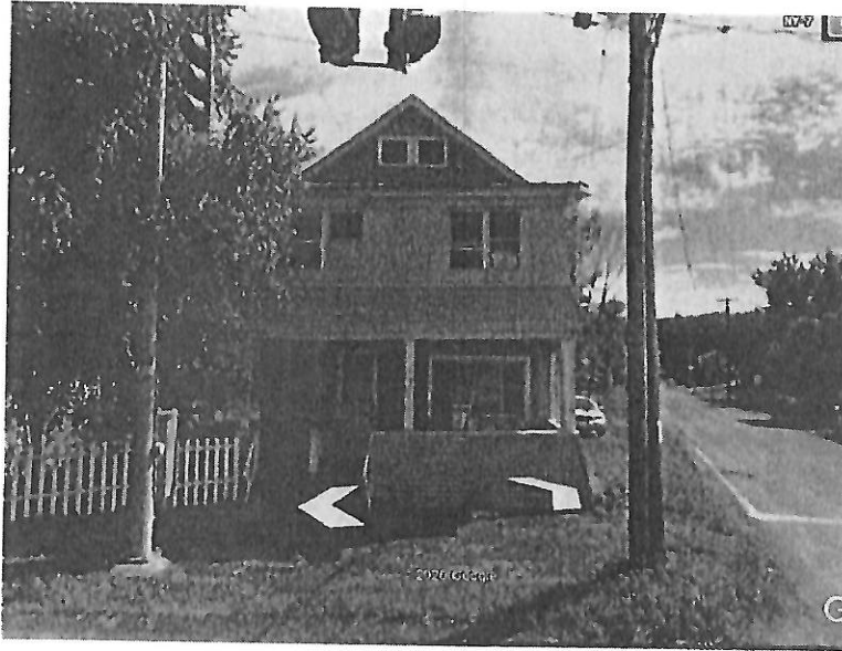
Before 12/29/19 Fire: 111 Darby Hill Road (Looking South)
