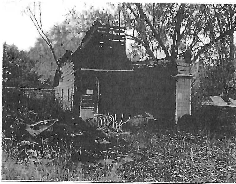
Remaining Outbuilding Structure, 10/22/2020 Looking East
