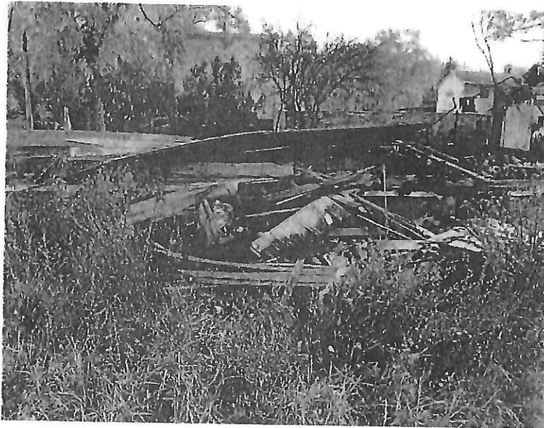
Remaining House Structure, 10/22/2020 Looking East
