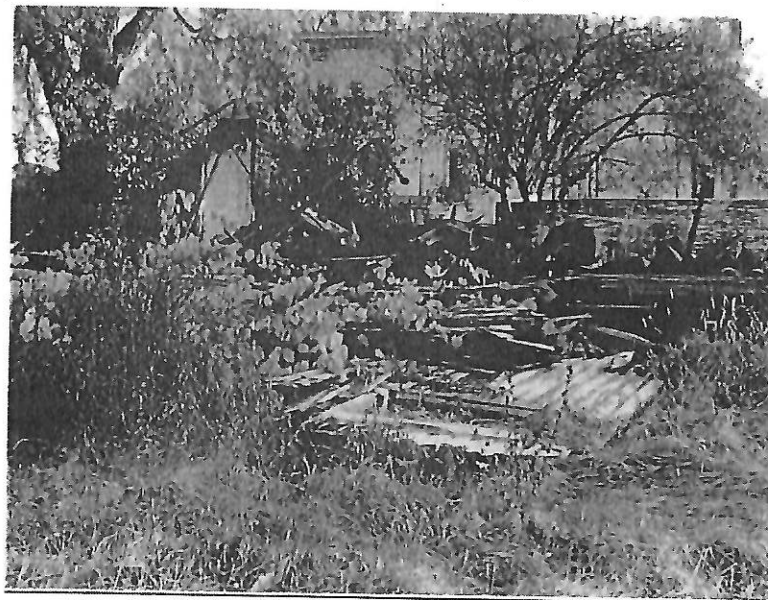
Remaining House Structure, 10/22/2020 Looking East
