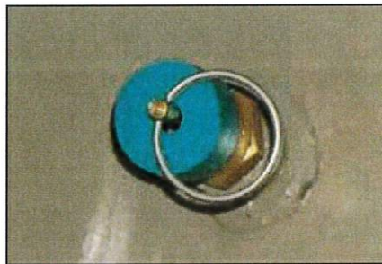
Figure 4. Automatic Pressure relief valve.
