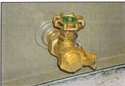
Figure 3. Drain valve with sampler.
